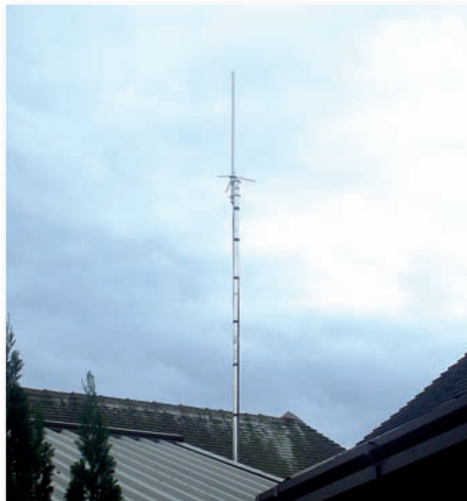
Pupils helped to assemble the new dual-band v.h.f./u.h.f. antenna that now adorns the end of their building.
